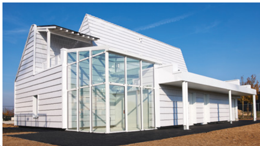
Architecte: BRUNO ROLLET
